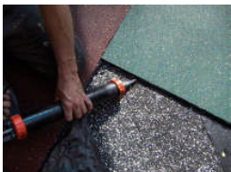
Apply Glue to bevel underside of tile.
